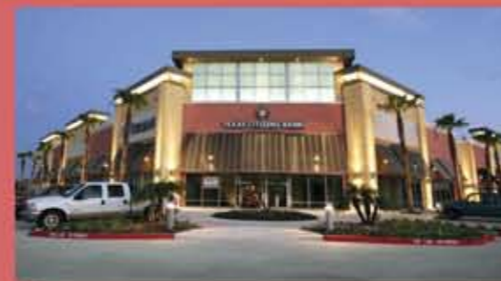
Retail Phase I – Ready for Occupancy
